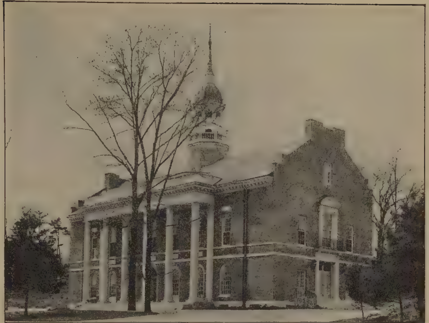
492 Bigelow and Wadsworth, architects; photograph by Thomas Ellison
